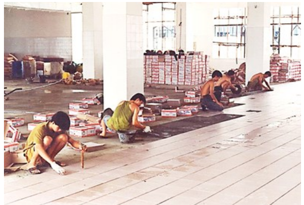
Tile Bonding & Waterproofing at Camel Nut Factory
