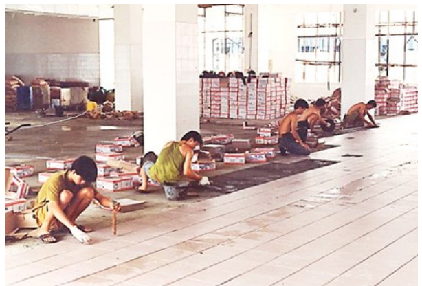
Tile Bonding & Waterproofing at Camel Nut Factory
