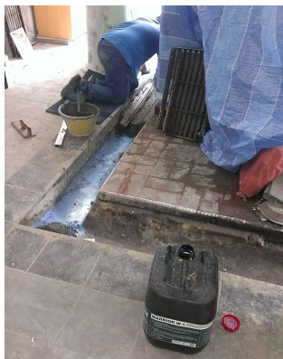
Re-surfacing the drain
