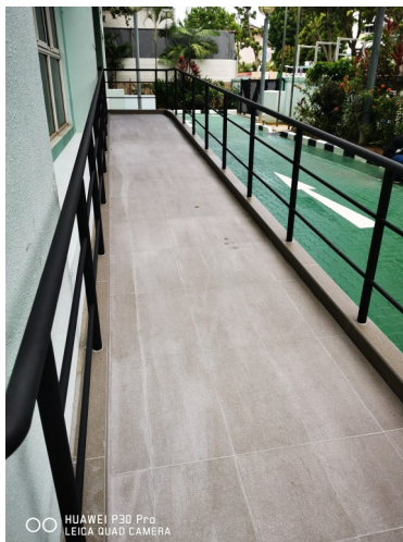
After treatment, free calcium may flow out from the cement joint. It can be removed by scrubbing. Suggest pre-treating the joint with SS10 before AS17 treatment.
