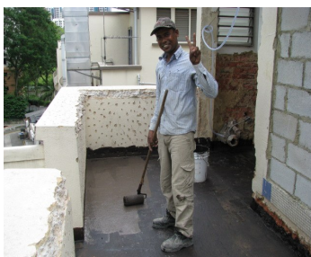
3 coats on the roof deck. Cured into non-tacky membrane.
