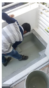
3 coats on the roof deck. Cured into non-tacky membrane.
