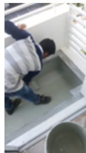
3 coats on the roof deck cured into a tacky membrane.
