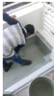
3 coats on the roof deck cured into a tacky membrane.
