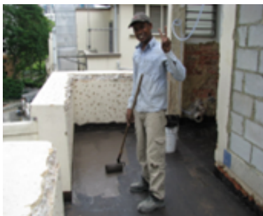
3 coats on the roof deck cured into a tacky membrane.
