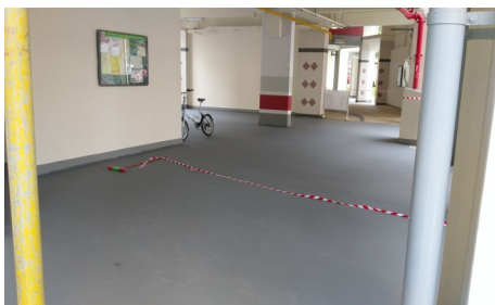
Floor Coating at HDB void
