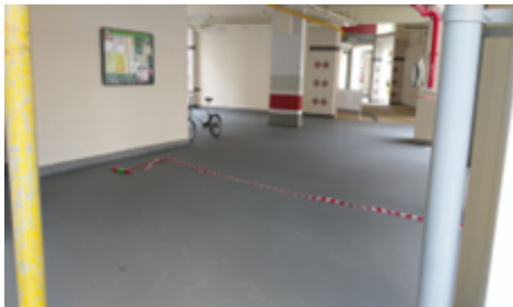
Floor Coating at Void Deck
