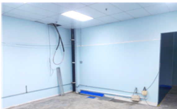
Walls coated with PU400
