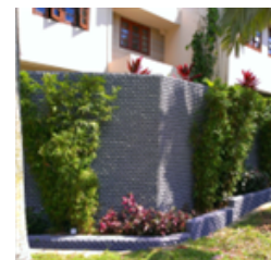
Used as coating on parapet wall
