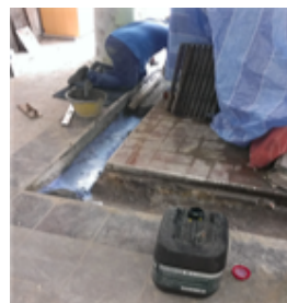
Re-surfacing of drain using W1
