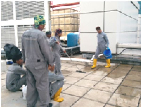
Sealing Roof Leaks - HP Alexandra
