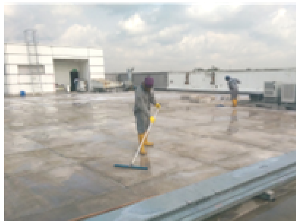
Sealing Roof Leaks - Motorola Building
